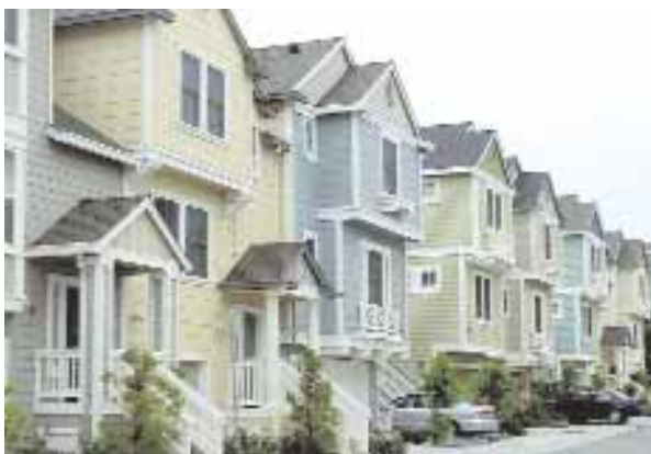
The city of San Mateo, in the greater San Francisco Bay Area, has had 189 affordable units built under its inclusionary housing program since 1996. The townhouses in the Classics at Humboldt Street development, completed in 2003, include a total of 25 two- and three-bedroom units. Three of these units are below market rate, affordable to households whose incomes do not exceed 80 percent of the area median income.
